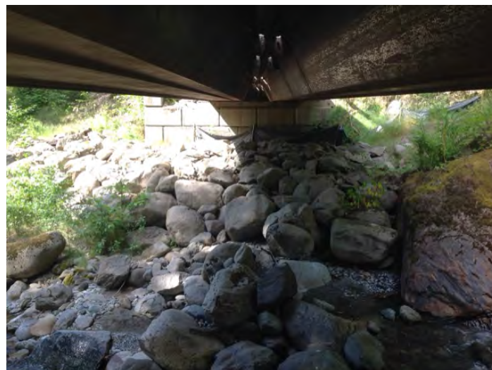
Right Bank Abutment when facing downstream
