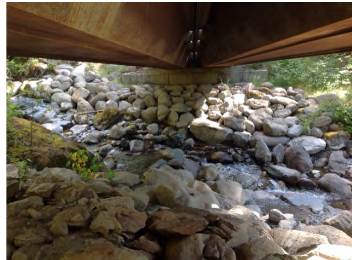
Left Bank Abutment when facing downstream
